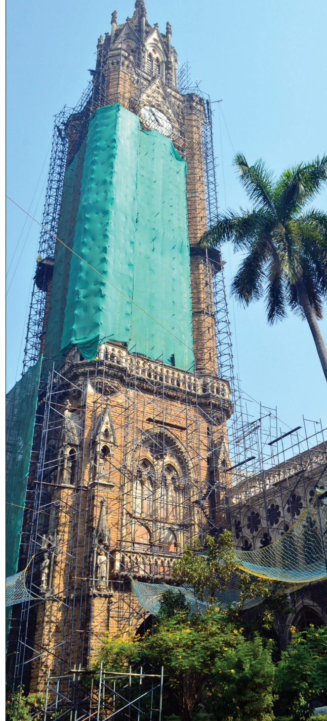
Above: an elaborate scaffolding structure was installed, to ensure that all elements of the building would be dealt with utmost care and also with consideration to the safety of the workers.
